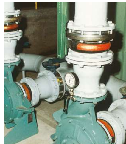
STENFLEX® type A-1 used at pumps
